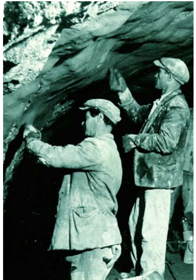
Impermeabilisation of Lötschberg (Switzerland) railway tunnel
