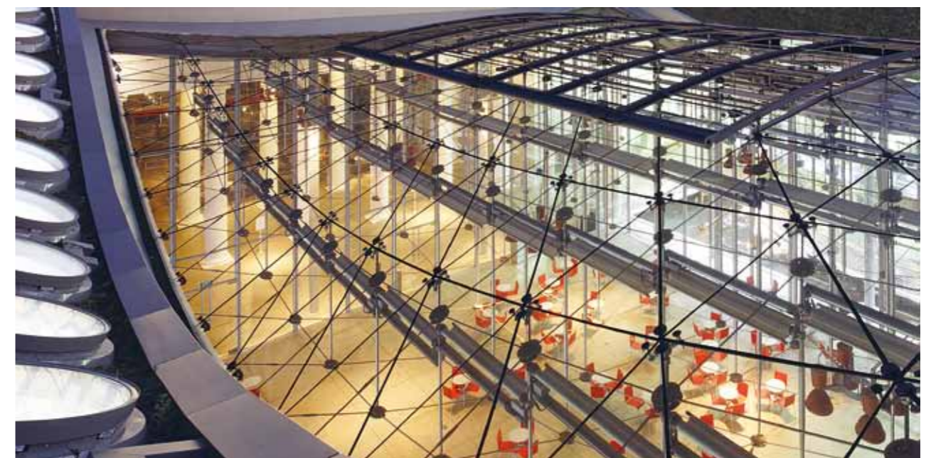
Superior: California Academy of Science, Exhibition and Research Center, San Francisco, 2008 Arquitectos Renzo Piano Building Workshop; Fachada Josef Gartner
